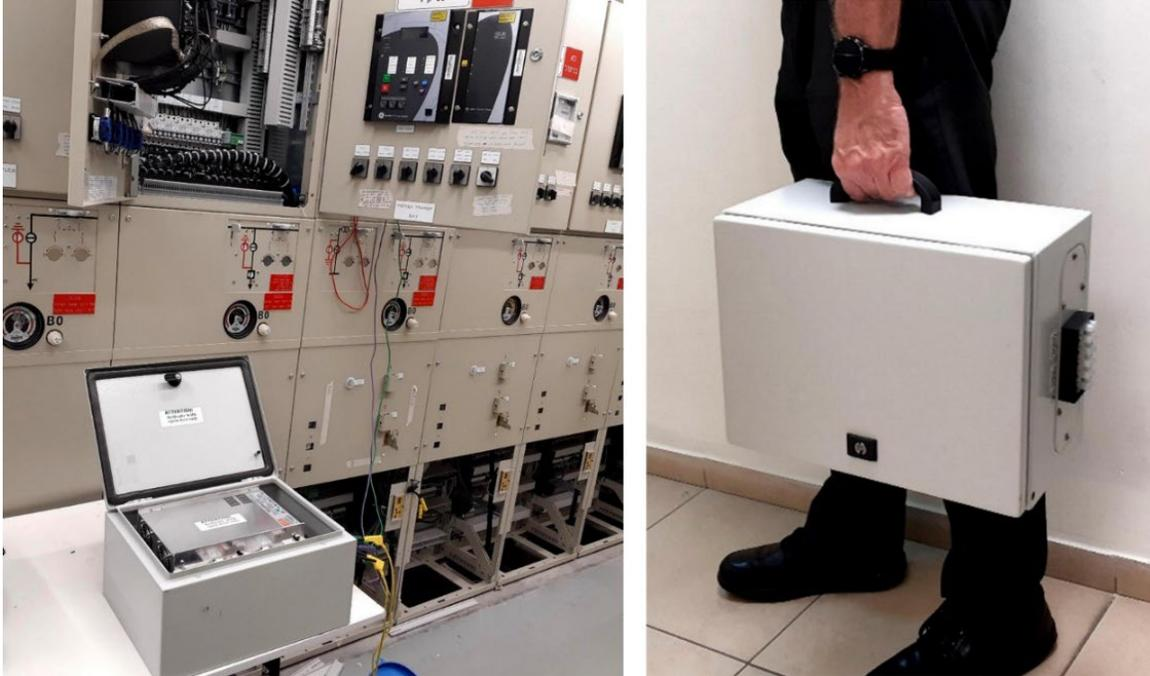
This compact backup power supply protected from HEMP and is capable of supply up to 25 A at 237V. The device is equipped with internal electronic protection against external short circuits and overloads. It is also equipped with a digital voltmeter and an ammeter for external circuit monitoring.
